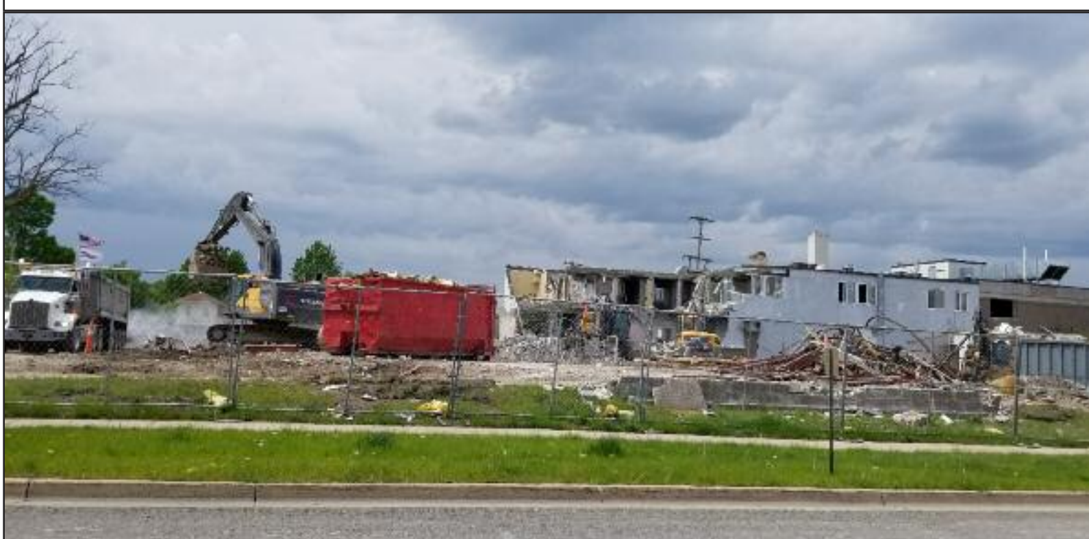
The walls of Kelsey Memorial Hospital are being reduced to rubble.
